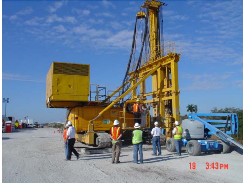
Photograph 3. The TRD machine, with the cutting post inserted into the ground. (Courtesy of Hayward Baker, Inc.)
