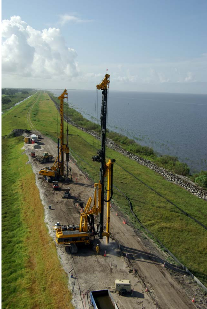
Photograph 4. CSM machine (foreground) with predrilling being conducted in the background. (Photograph courtesy of Coastal Caisson Corp.)
