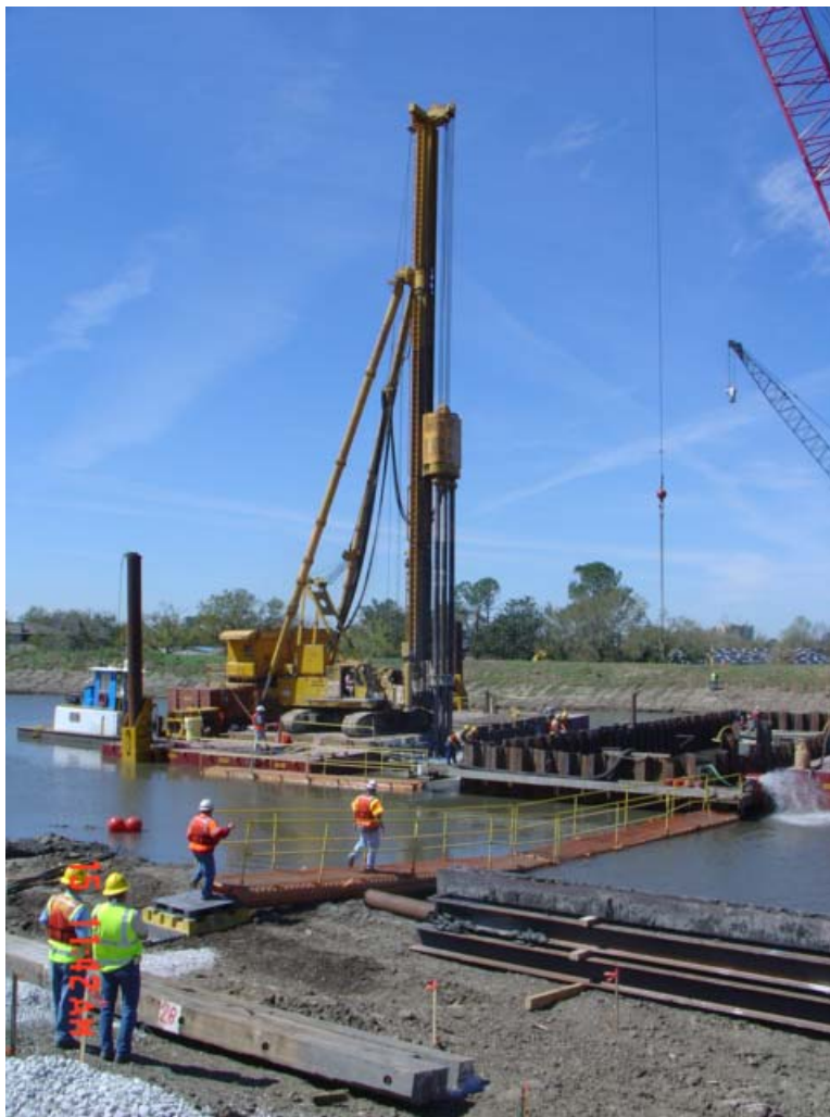
Photograph 1. DMM machine (triple axis) operating in river conditions (Courtesy of Raito Inc.).
